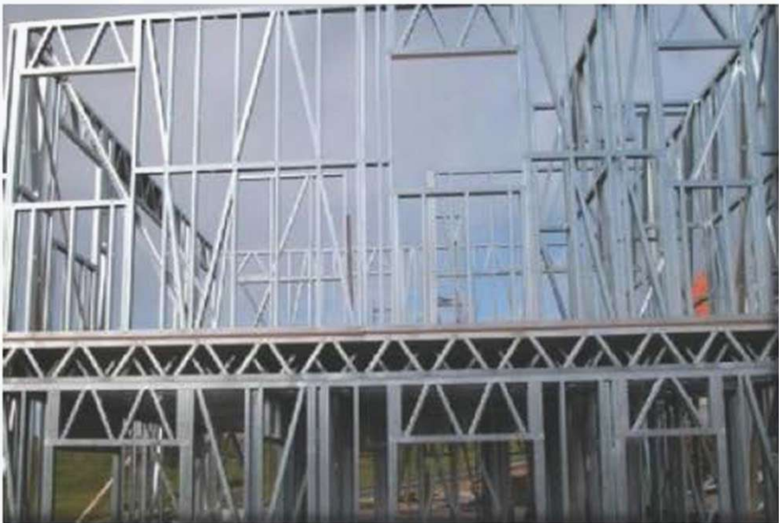
ASSEMBLED TO ERECT STRUCTURE
